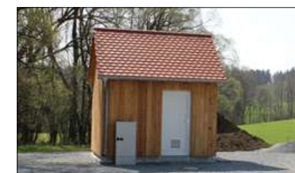
Example: Installation in a machine house
